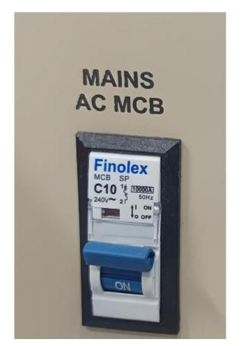
**Step 7**: - Switch ON AC supply/Grid/Mains switch and check at display mains LED indication and also at LCD representation.
